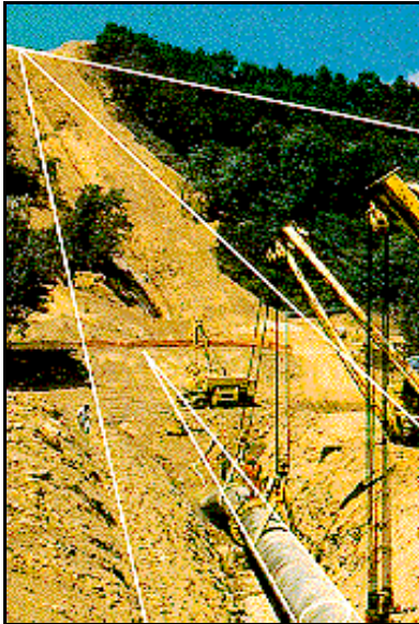
Figure 1: Installation of a typical
