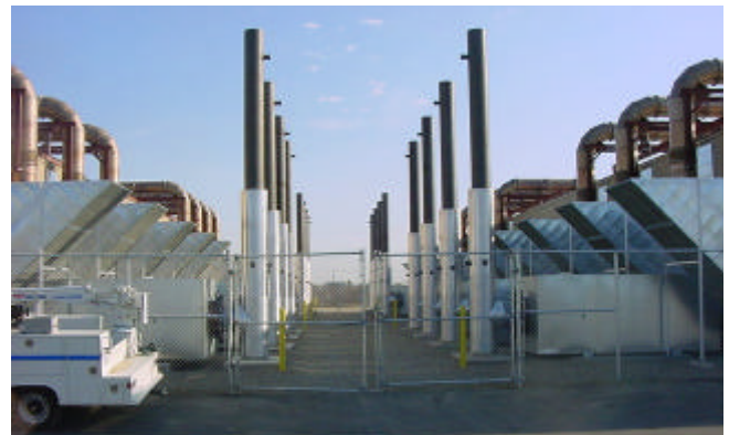
View Between Engine Buildings
