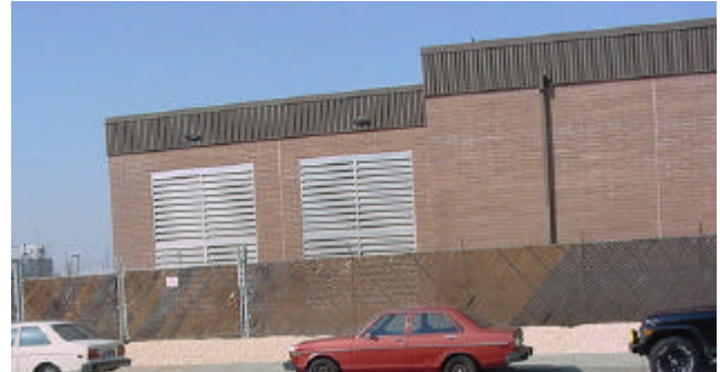
Standby Generator Building
