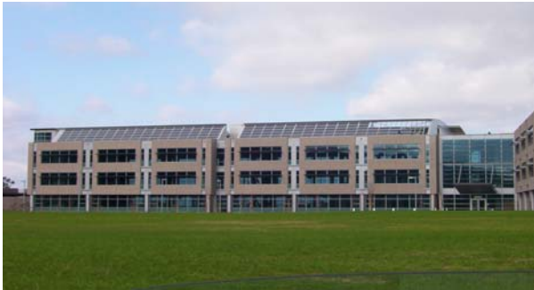
Roof Mounted Fixed PV Array providing Power and Architectural Accent
